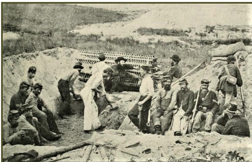
FEDERAL TROOPS EXTEND THEIR TRENCHES ON MORRIS ISLAND DURING THE SIEGE OF FORT WAGNER. A MOVABLE SAP ROLLER IS USED TO PROTECT THE MEN OF THE 1ST NEW YORK ENGINEERS AS THEY WORK.
